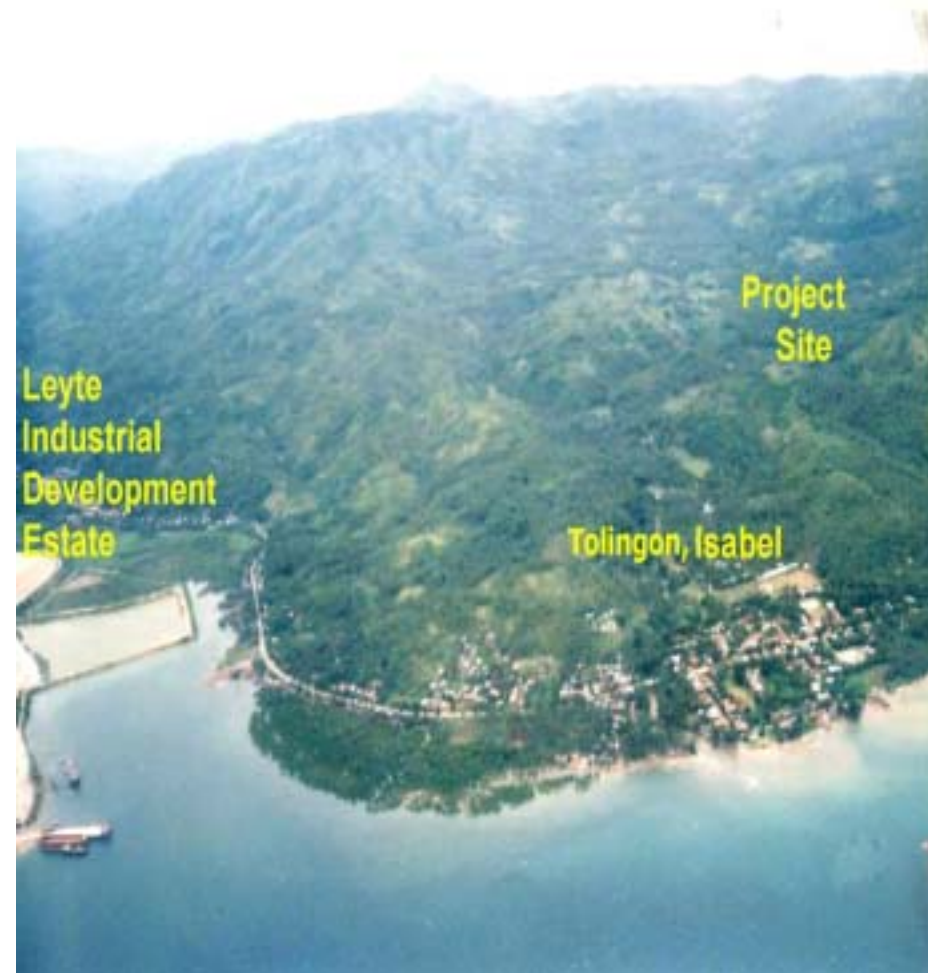
Aerial view of the Cement Project
